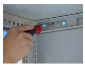
Inside fixation by nuts to avoid accident
